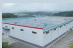
At our Western Japan logistics Center (Miki City, Hyogo Prefecture), we are operating a mega solar project with solar panels on a portion of open land and on some of the roof space of the center itself.
